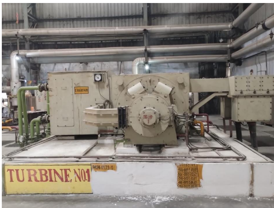
Figure 3: Turbine extraction cum bleed condensing
